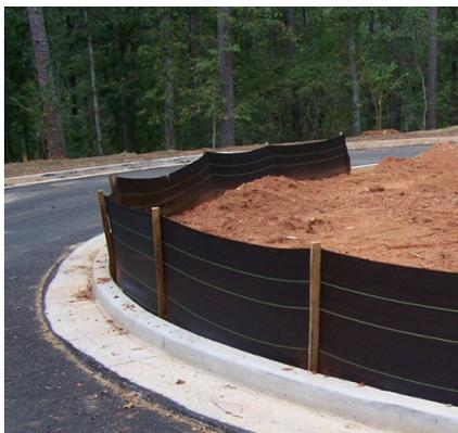
**Silt fencing and BMPs limit runoff and erosion during site disturbance.**
