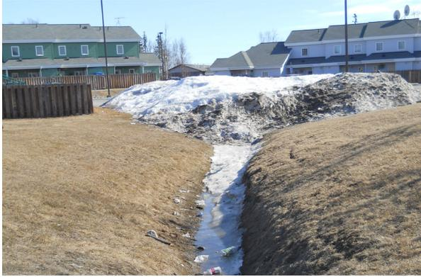
*When best stormwater practices are used, such as this snowstorage treatment swale, it can reduce public costs from offsite drainage and water quality problems.*
