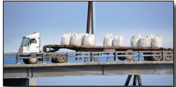
Each supersack of cement weighs 3,300 pounds. Cranes on the ship hoisted twelve sacks onto each flatbed. The loads left the dock about every seven minutes and made their way to a warehouse up the hill.
