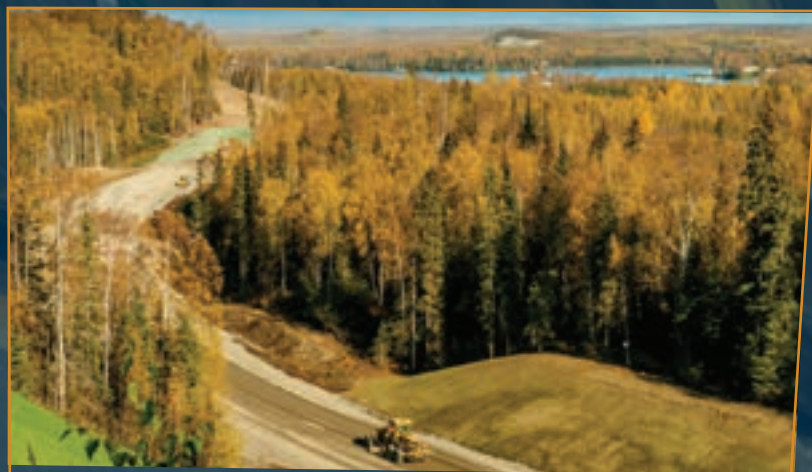
South Big Lake Road Realignment: $9.7 million, built new segment of two-lane gravel road from east of Jade Lake to Burma Road & Susitna Parkway intersection.
