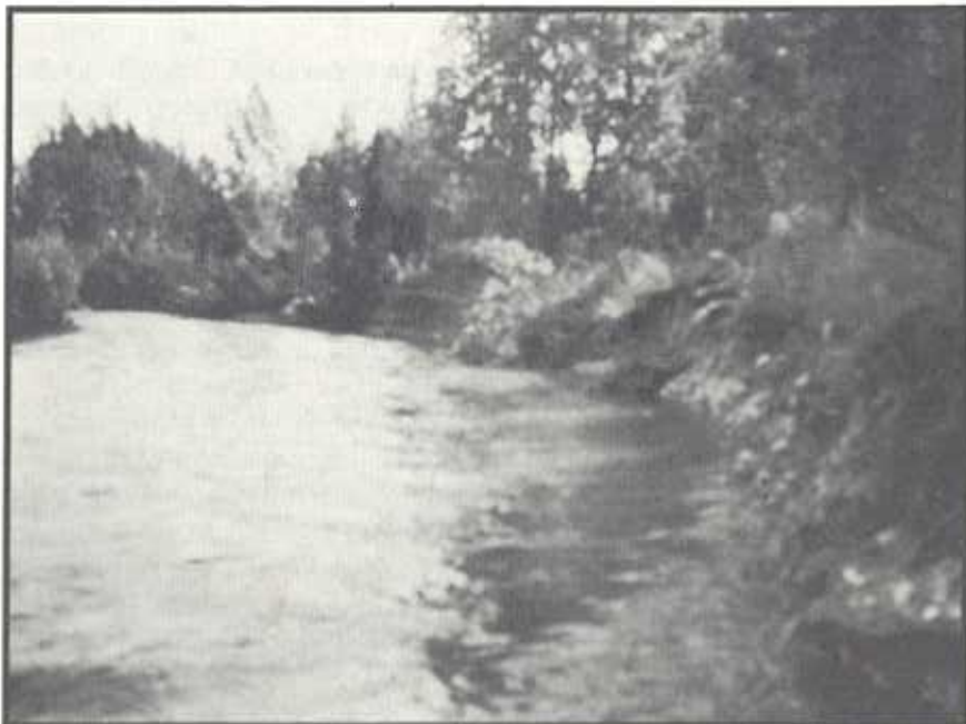
Example of stream bank erosion.
