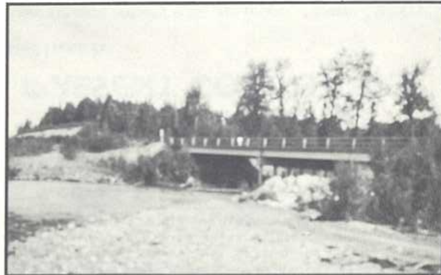
Troublesome Creek at Parks Highway bridge.
