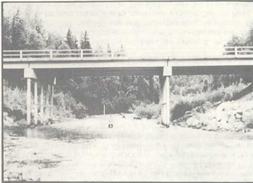
Looking upstream on Byers Creek at Parks Highway Bridge.
