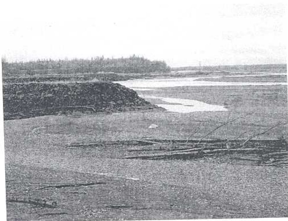
Photo 6 – Looking downstream at spur dike 2 from spur dike 1.
