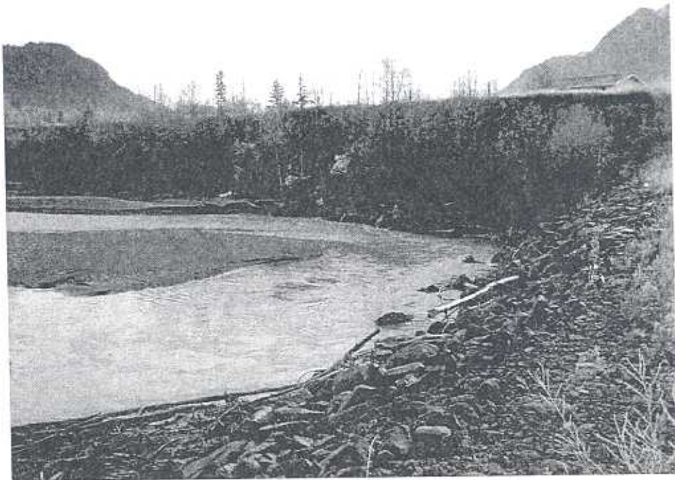
Photo 4 – View looking upstream from spur dike 4 at area where low flow impinges on bank between spur dikes 3 and 4
