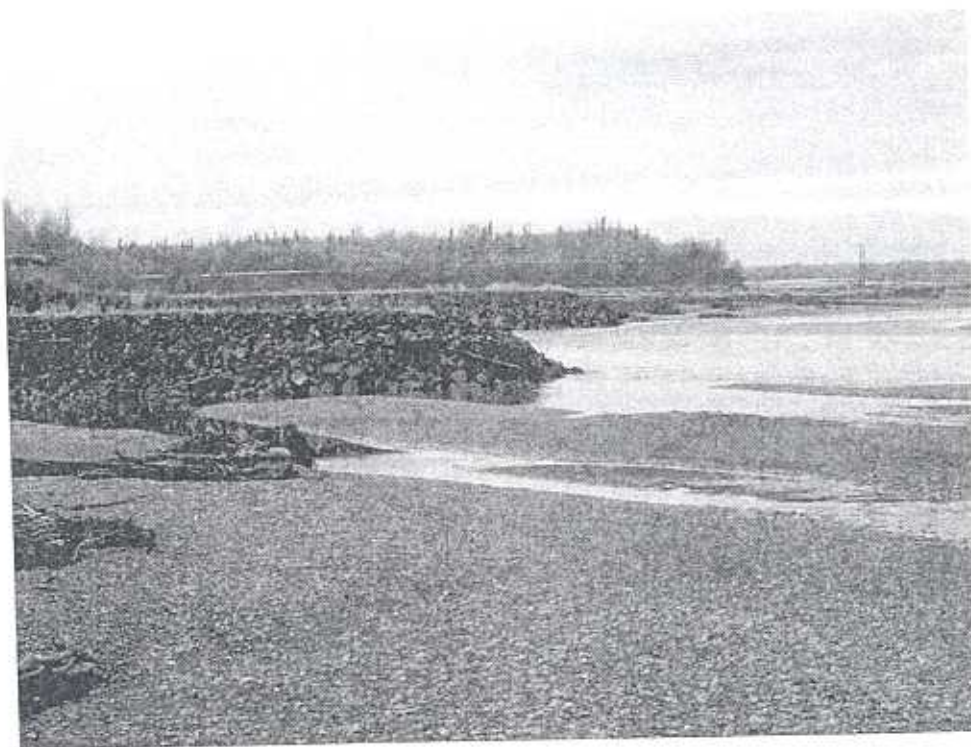
Photo 5 – Looking downstream from spur dike 2 at spur dikes 3 and 4.
