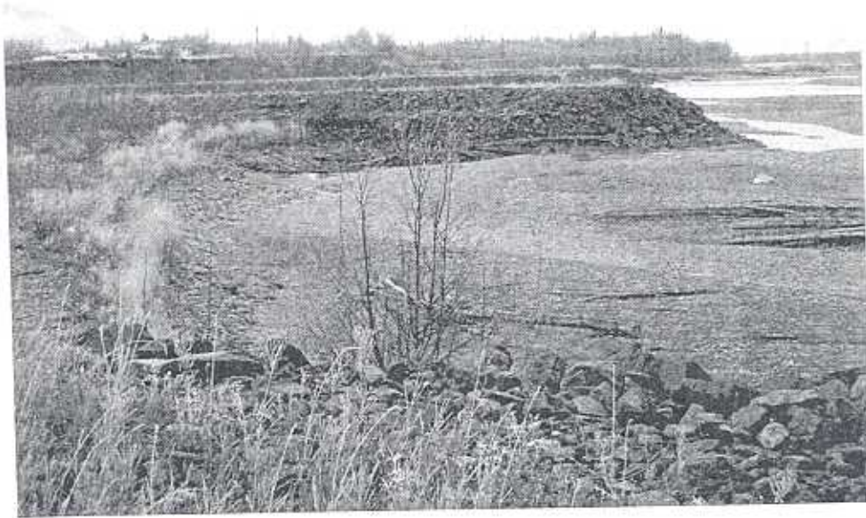
Photo 7 – Looking downstream at area between spur dikes 1 and 2 from spur dike 1, higher vegetated deposits indicate main flow has not recently reached the bank in this area
