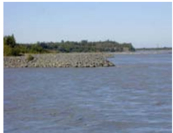
Spur Dike on the Matanuska River
