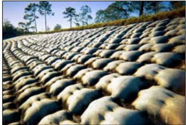
Concrete filled Mat
