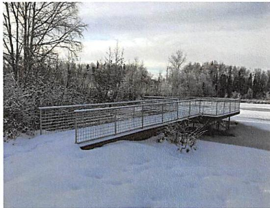
*Above photo: New platform with handrail structure and mesh pedestrian panels*
