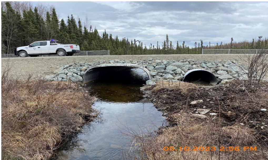
Above photo: New Fish Passage Culvert and Overflow Culvert
