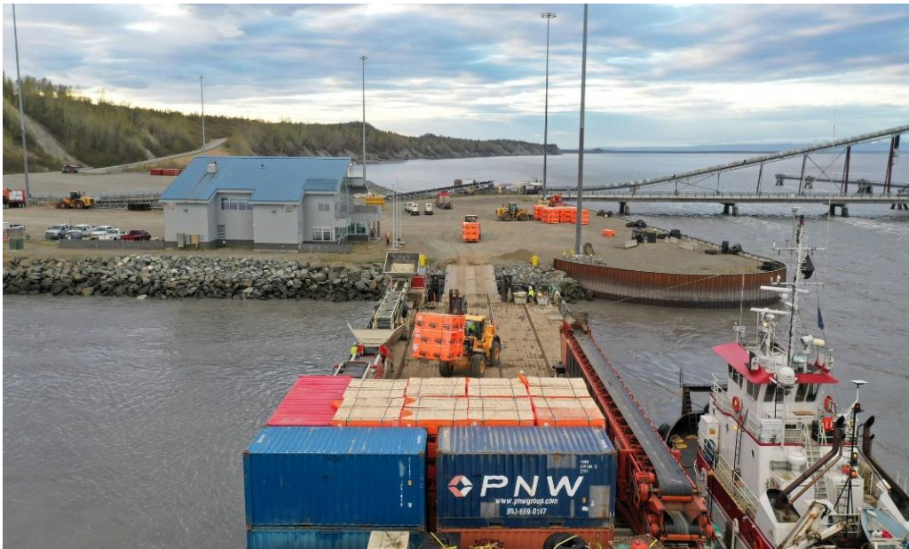
Above photo: Cruz Construction loading the Atlas
