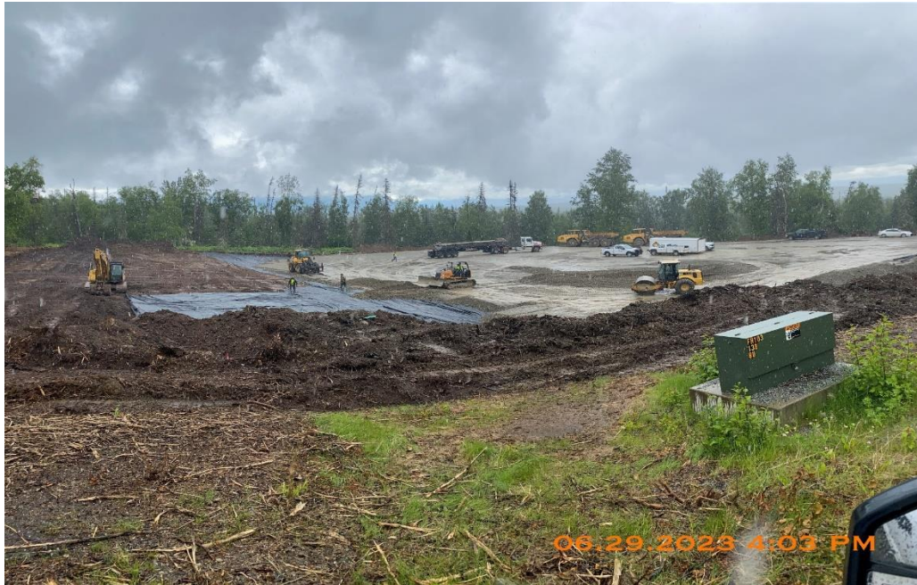
Above photo: GPRA Overflow Parking Lot Construction
