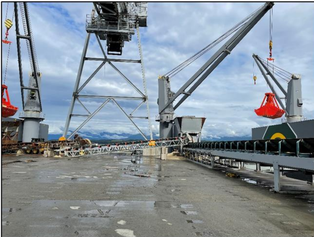
Above photo: Conveyor in operation on the trestle.
