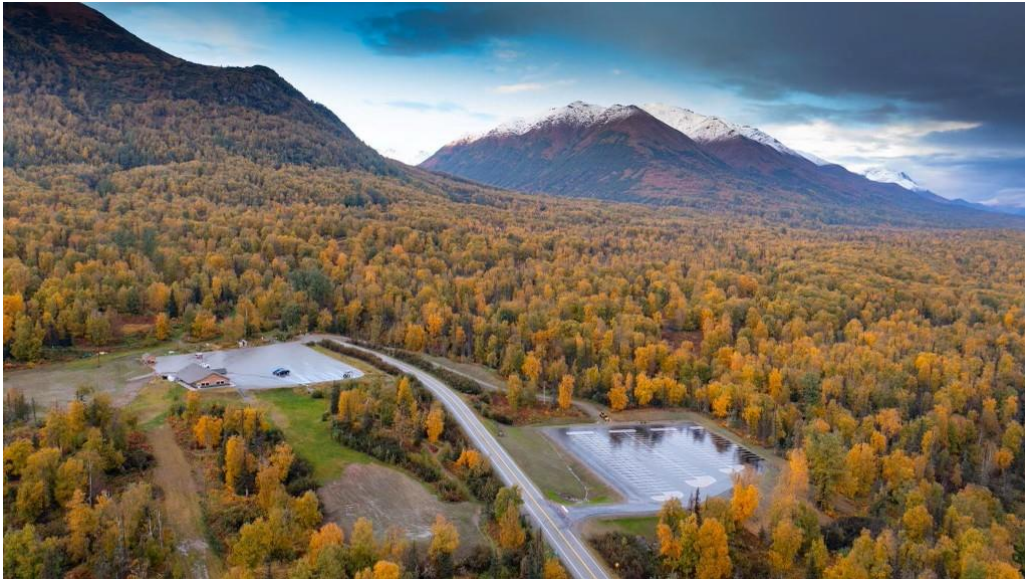
Above photo: GPRA Overflow Parking Lot After Construction
