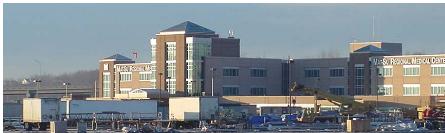
Construction of Mat-Su Regional Medical Center (Sandra Petal, MSB)
