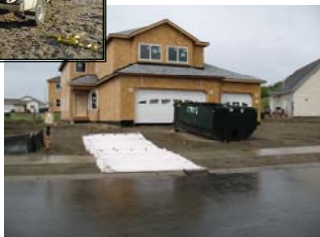
RESIDENTIAL CONSTRUCTION ENTRANCE
