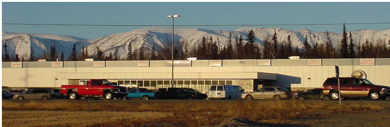
Retail Development, Palmer-Wasilla Highway (Sandra Petal, MSB)
