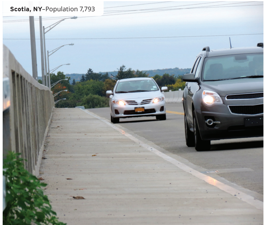
This sidewalk was installed over the existing bridge deck during a rehabilitation project.
