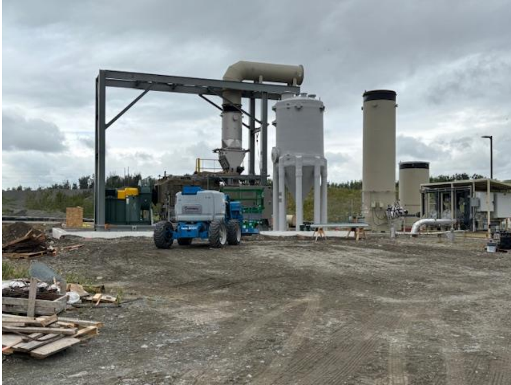
Photo: Leachate evaporation system under construction (June 2025)
