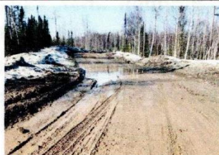
Mile Post y.y. A serious but very common drainage problem that is VERY common on our roads. This can probably be accomplished under an "extra work" item under the Maint. Contract. This may or may not require a CMP. Typically, a maintenance contractor doing this type of maintenance work will have the equipment and experience to make this type of repair. This road has been accepted for maintenance and I would think there is an obligation on the boro's part to provide an acceptable level of maintenance for safer and reasonable travel.
