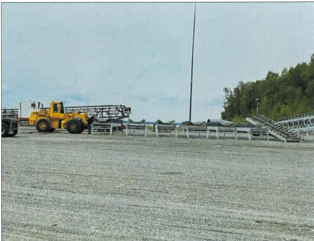
Conveyor Removal and Reconfiguration
