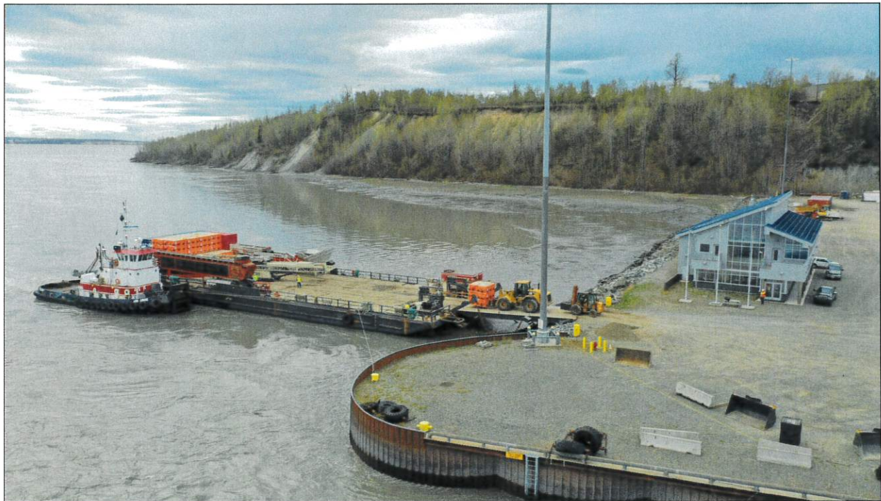
Cruz Construction Barge – Atlas
