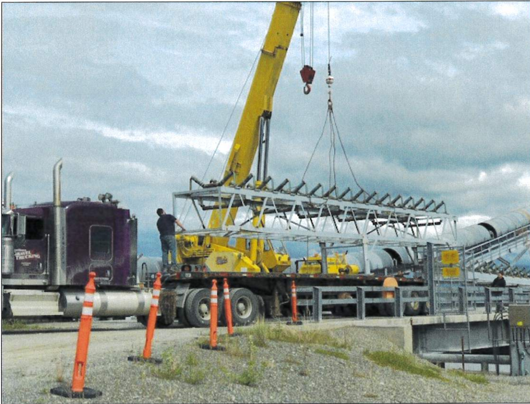
Conveyor Reconfiguration and Assembly
