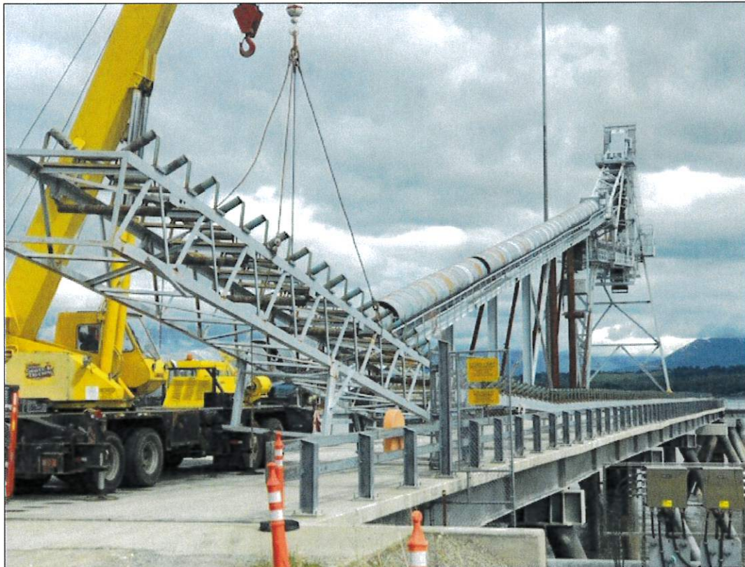
Conveyor Reconfiguration and Assembly
