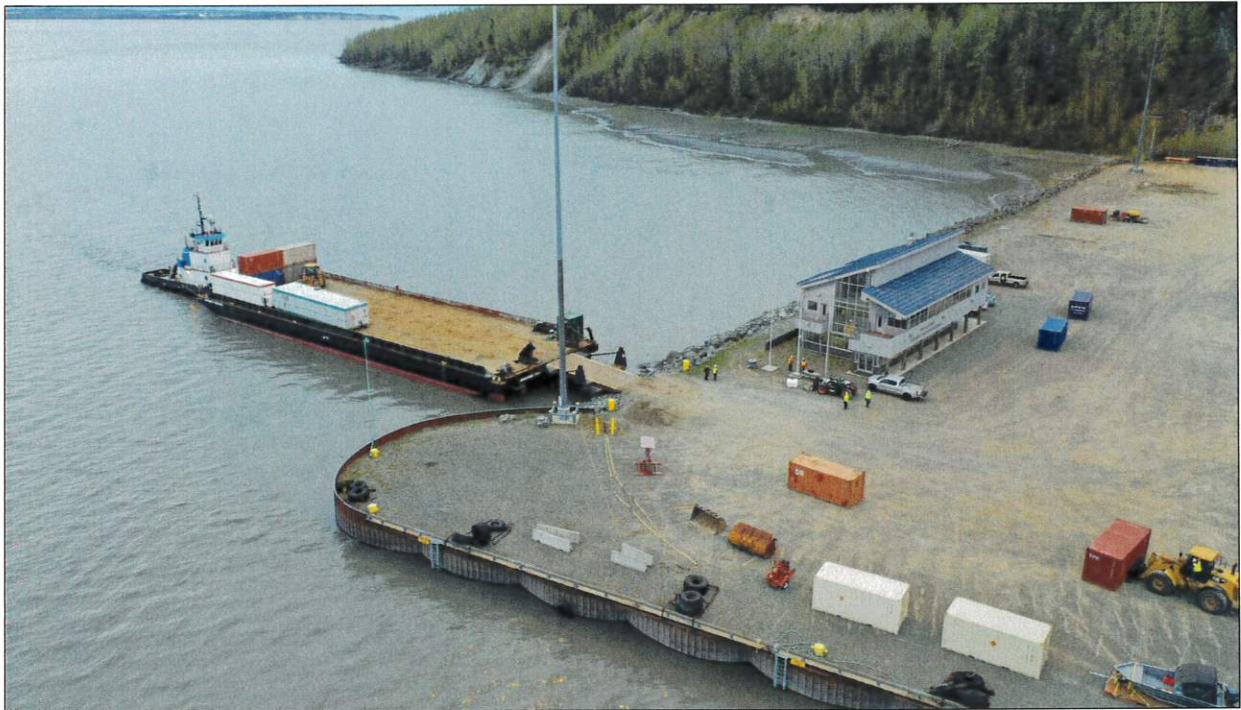
Cruz Construction – Baranof Provider
