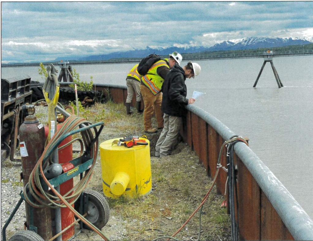
Barge Dock Repair – Cell 1
