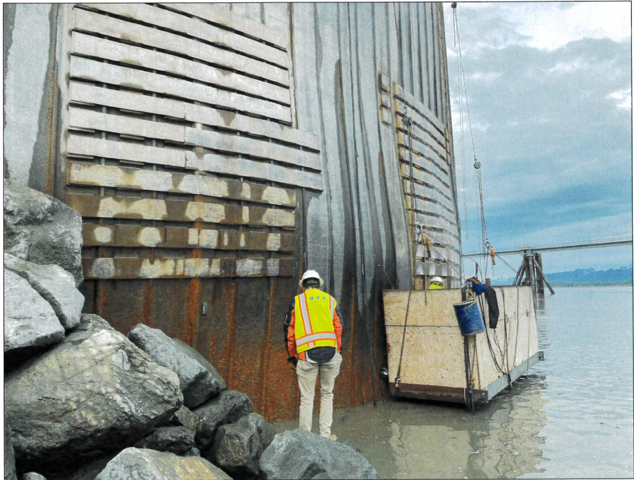
Barge Dock Repair – Cell 1
