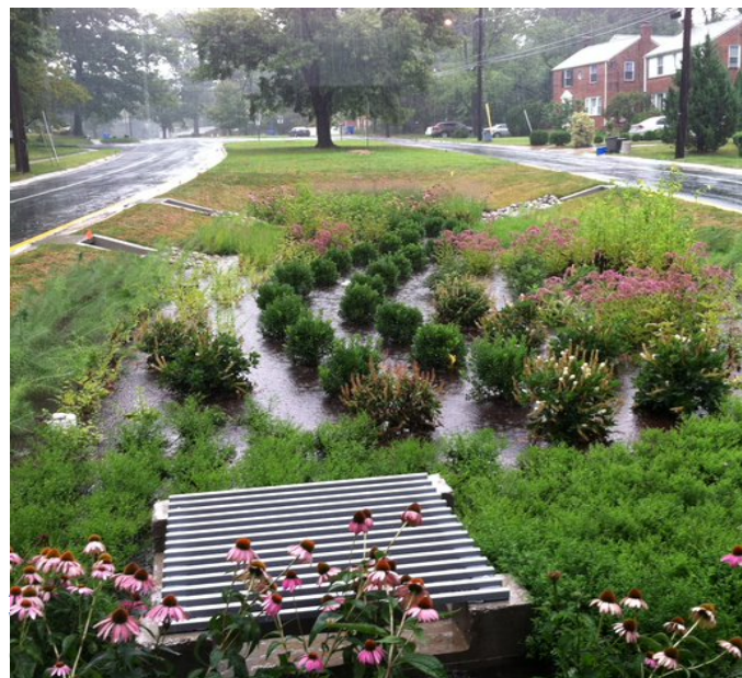
A bioretention practice in a suburban road median, capturing stormwater during a rain event.
