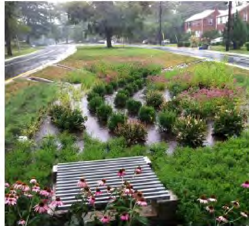
A bioretention practice in a suburban road median, capturing stormwater during a rain event.
