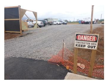
A construction entrance stabilized with gravel over filter cloth reduces the amount of sediment transported off site. Photo Credit: PG Environmental for USEPA
