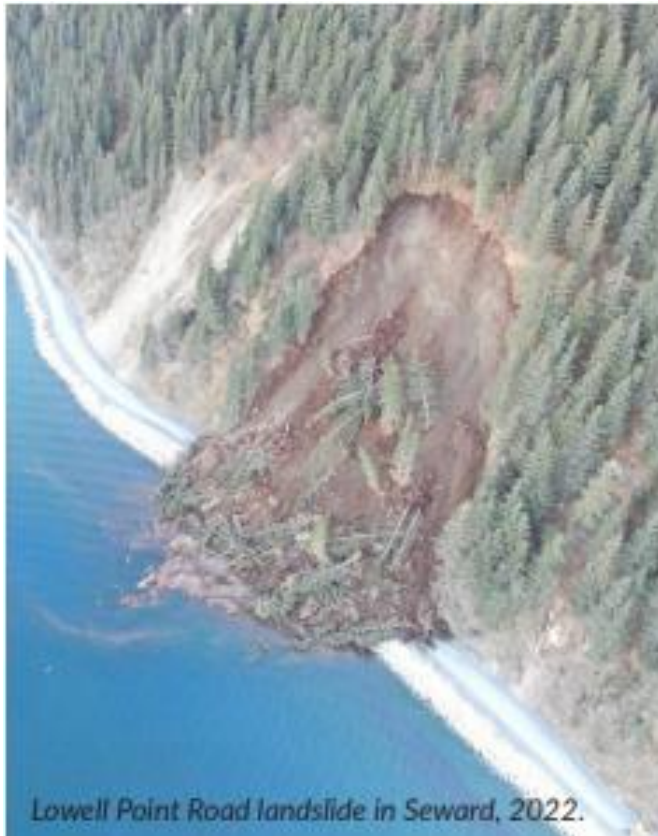
Figures 48: Landslide at Lowell Point, Seward, AK
