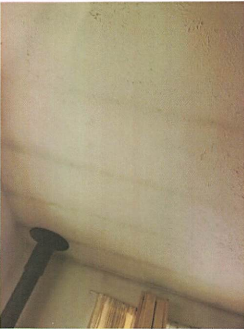
North ceiling with the mold marks and in the corners where it looks to have moisture accumulation.
