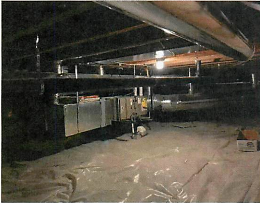
Crawlspace Forced Air Heat System
