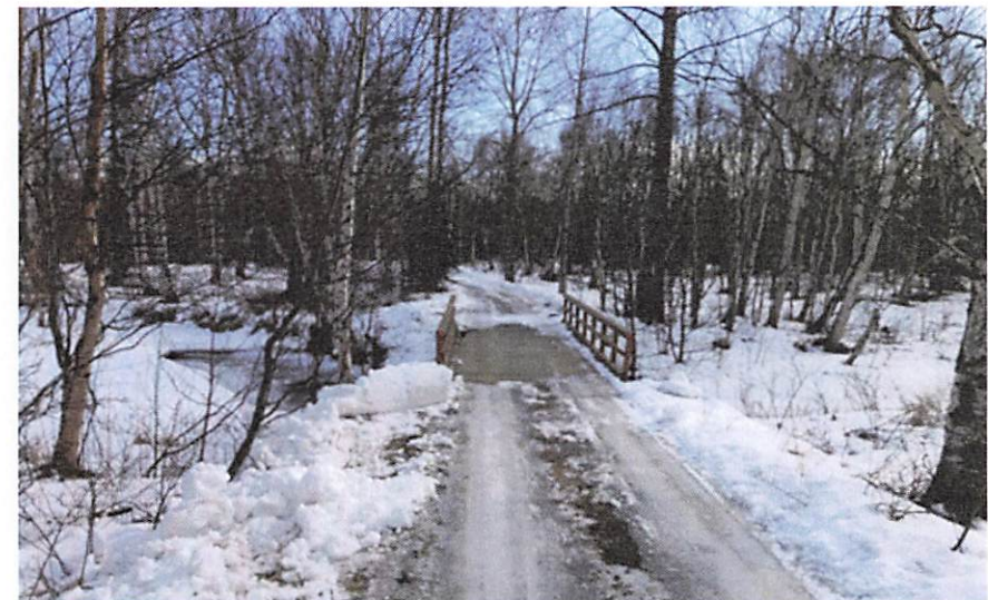
Subject Bridge Crossing Wasilla Creek
