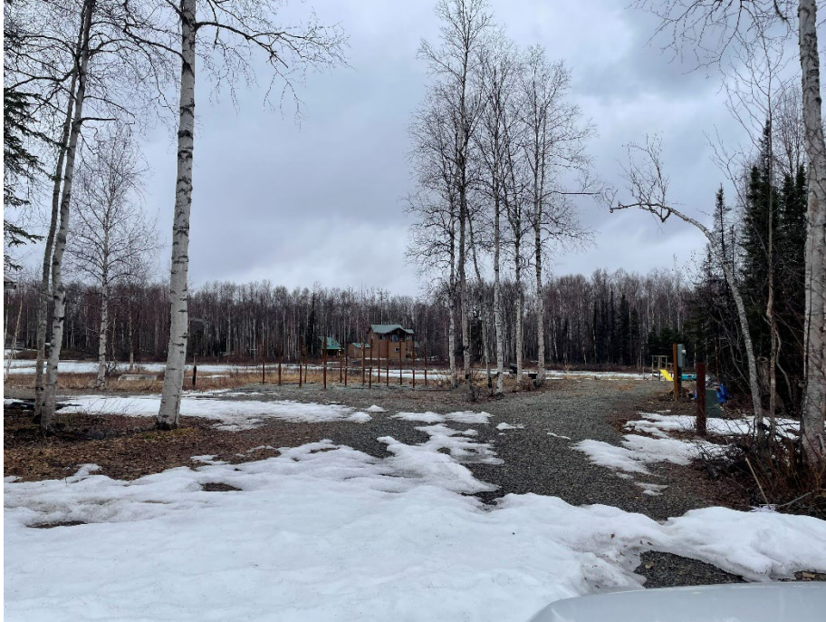
Looking from road to like. Can see foundation of structure started.
