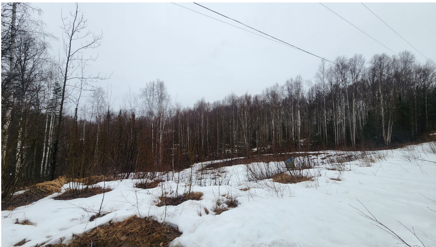
On subject property. Facing northeast along utility easement.
