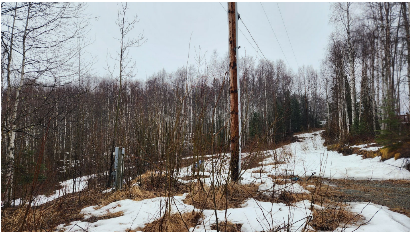
On subject property. Facing east along utility easement.
