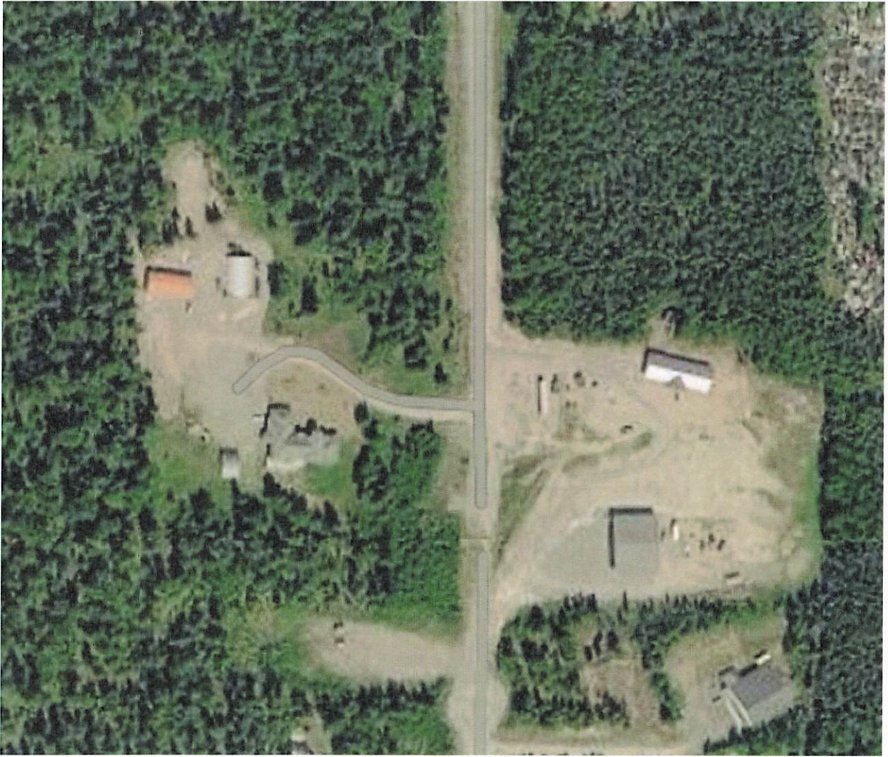
Figure 24 The gap has a hill in place and is impassable
