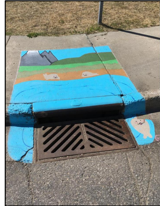
Inlet Artwork in Fairbanks. Image source: https://www.fairbanksalaska.us/engineering/page/storm-water-management
